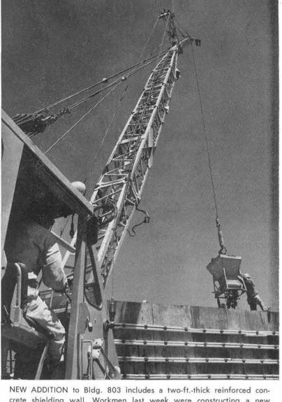
crete shielding wall. Workmen last week were constructing a new radiation effects laboratory to the Van de Graaff building used by Radition Physics Department 5310. The new lab will contain 2100 sq. ft. A 296-sq.-ft, service area for the building is also under construction. Plant Engineering Department project engineer is V. E. Kerr. (4543-3). Completion of the project is expected in early September.
